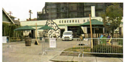
A former autobody repair shop is now home to three separate businesses, including a restaurant and brewery. Outdoor spaces are also an important aspect of the adaptive reuse of this building.
